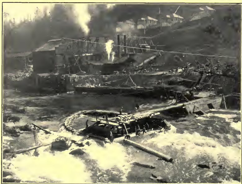
CONSTRUCTING DAM ABOVE SNOQUALMIE FALLS.
